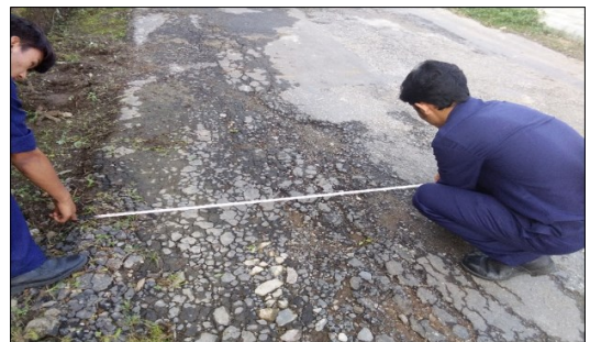
Fig. 5. Alligator Crack
